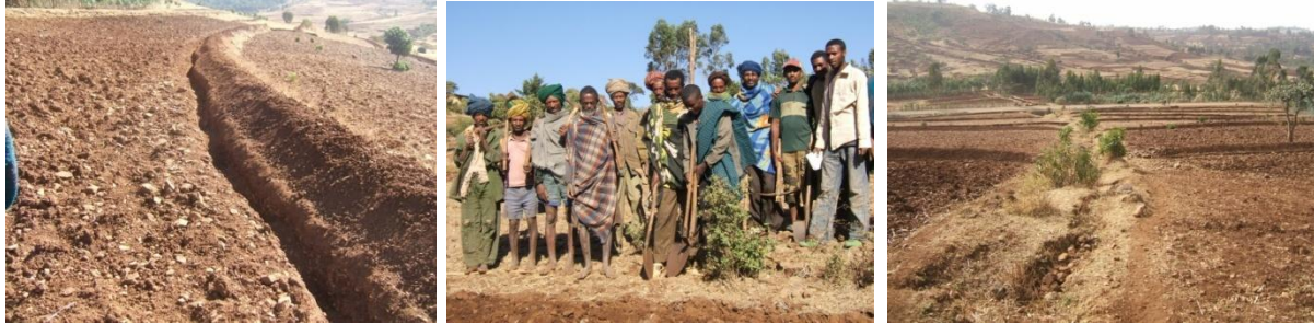
Photo 4. Bunds and waterways constructed in 2011/12
